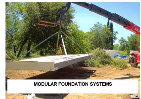
ON-SITE PREFABRICATION
