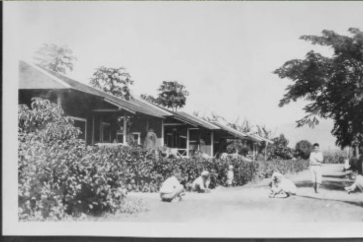
Ewa Plantation Company Laborer's Village
