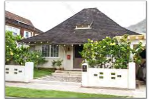
C.W. Dickey Residence 3030 Kalakaua Avenue
