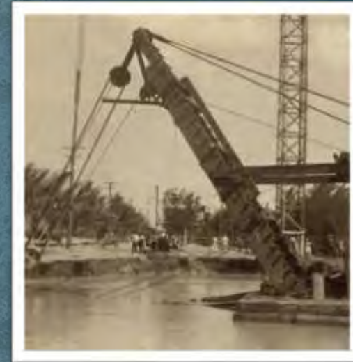
Dredging of Ala Wai Canal
